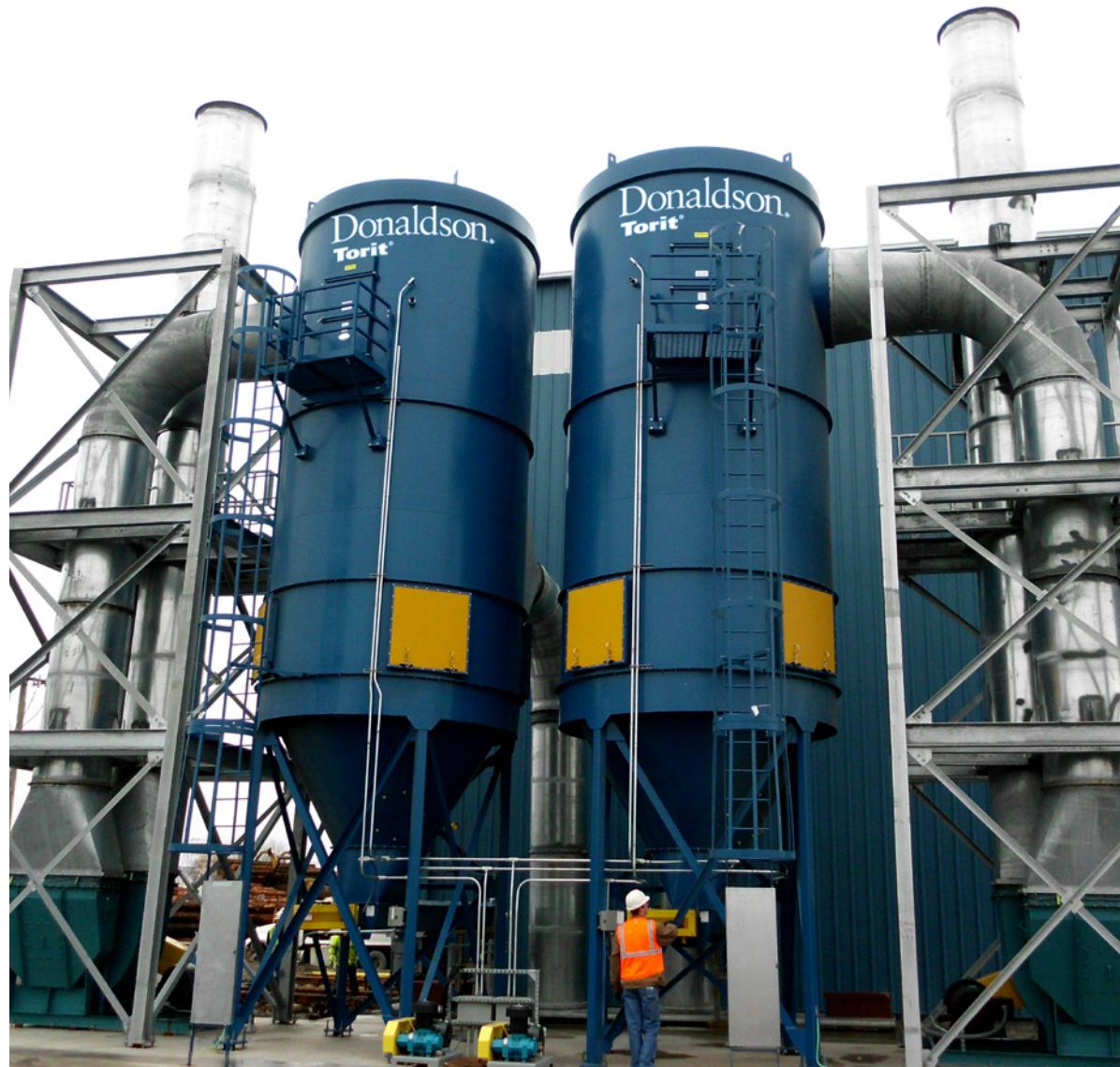
Figure 2. Traditional Centralized Baghouse Collectors
