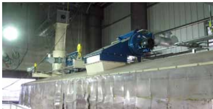
Dust collectors with fluted filter packs are much smaller than conventional dust collectors, which allows the collector to be integrated into a truck load-out hood.
